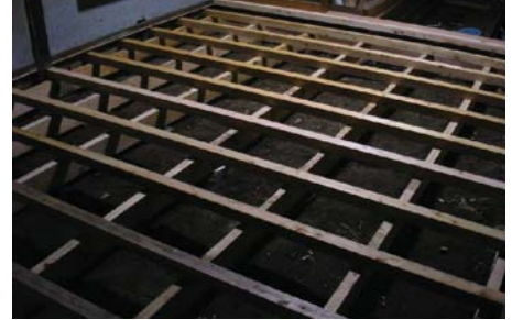
24.02.2005: Then the secondary loadbearing structure
