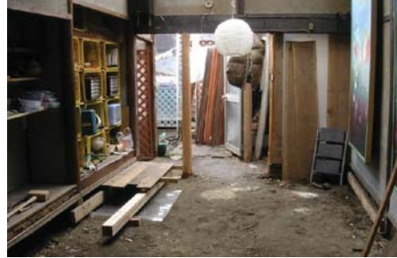
10.02.2005: Central room after cleaning up
