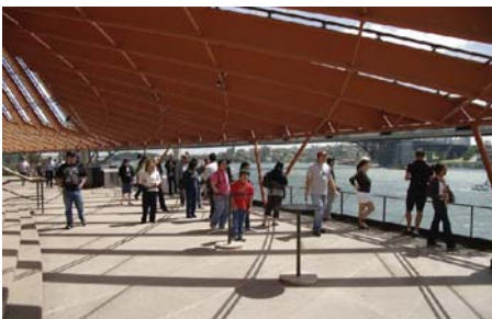
Picture 12 Overlooking harbour and Harbour Bridge
