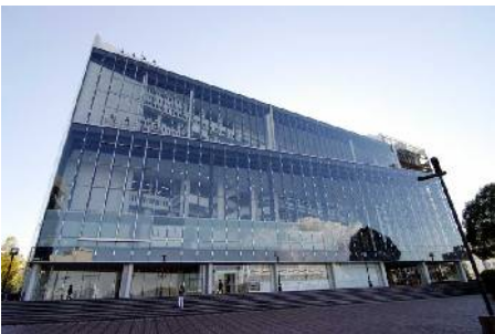
15 – Paint House Building
