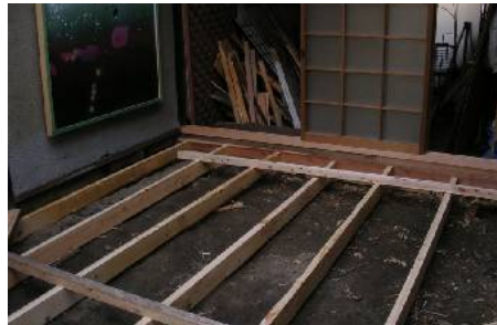
23.02.2005: Next came the primary loadbearing structure for the floor
