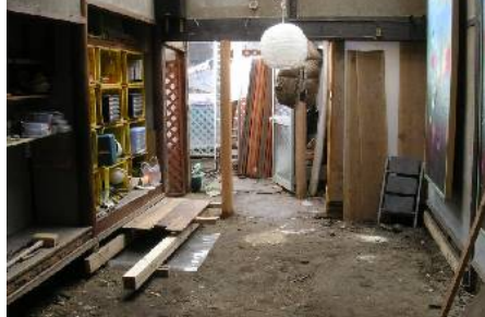
10.02.2005: Central room after cleaning up
