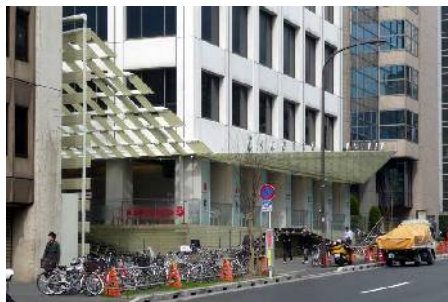
7 – NTT Aoyama Building Renovation
