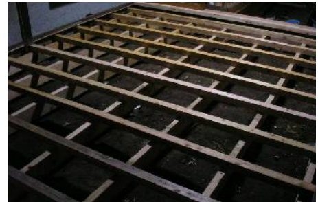
24.02.2005: Then the secondary loadbearing structure
